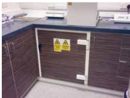
Figure 10: Smooth, easy to clean surfaces are appropriate in view of the risk of a radioactive spill. Radiation warning signs denote potential hazards
