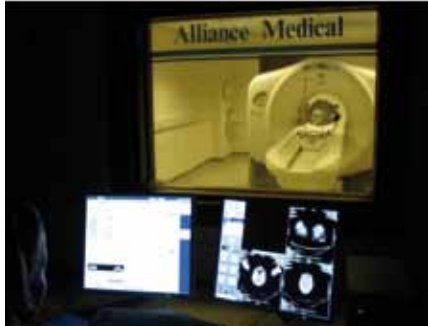
Figure 13: Control room where shielding with lead salt glass and lead bricks is used in the adjoining wall to the scan room
