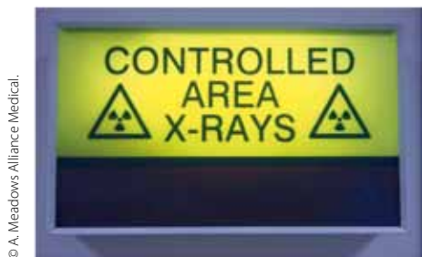
Figure 16: External flashing radiation warning sign during CT x-ray exposure
