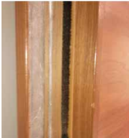
Figure 14: Side view of the scan room door. Lead lining approximately 4 mm wide can be seen and provides additional shielding
